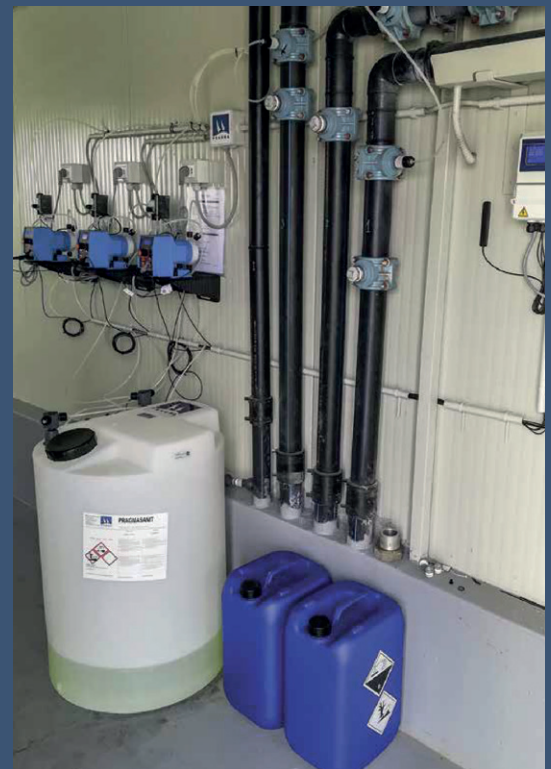
Stabilised chlorine dioxide dosing system with activator and protective film for sanitary water, with data communication and error reporting system via Ethernet module.
